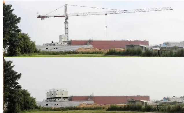
Figure 12: View of the SPIRAL2 phase-1 building construction (July 2013).
